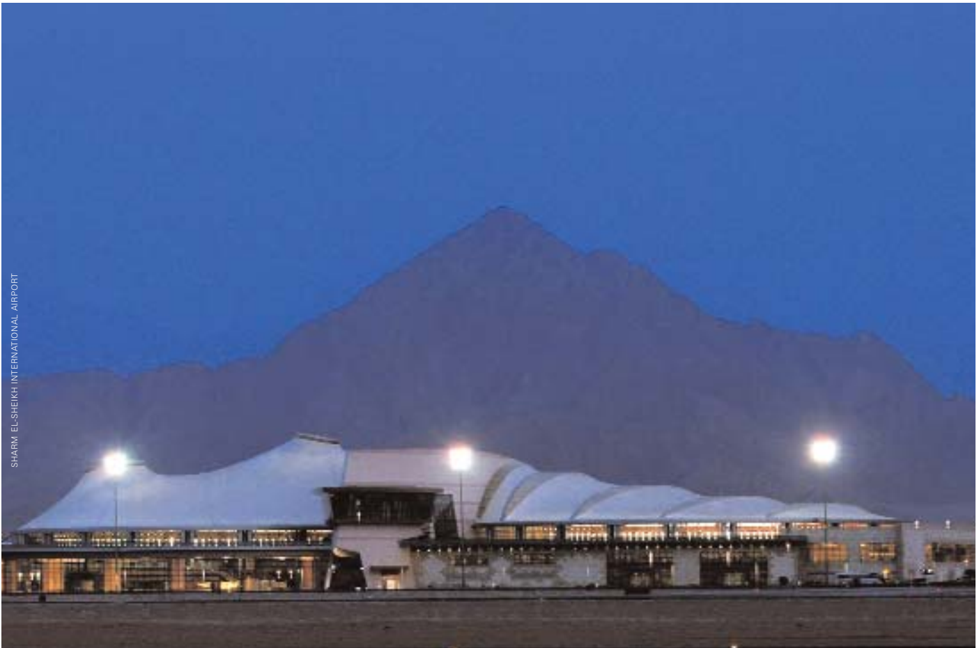
The new two-level, 43,000-square-meter Sharm El-Sheikh International Airport terminal features 40 check-in counters and one domestic and six international gates. The building's architectural design marries two circular-shaped halls to a central hub that serves as the passenger transit area.
